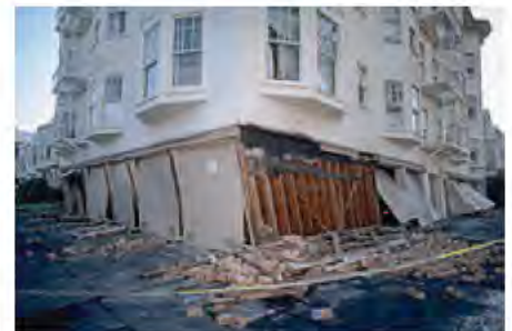
A building in the Marina District at Beach and Divisadero settled onto its buckled garage supports during the Loma Prieta Quake.
