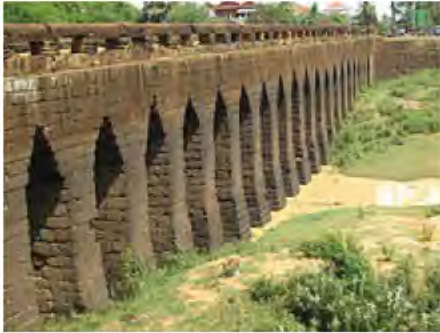
The Khmer Empire's bridge of Spean Praptos, a corbel bridge in Siem Reap Province, Cambodia.
